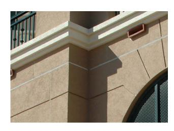
All butt joints, intersections and ends shall be caulked at the time of installation using an elastomeric sealant, such as Plastic Components' Ultra-Tech™ (PC-ULTW).
