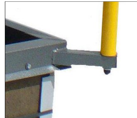
Rail Supports are Welded to Curb
